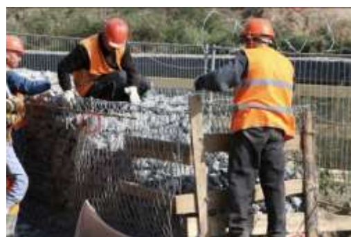
Fig. 3. Gabion structures
