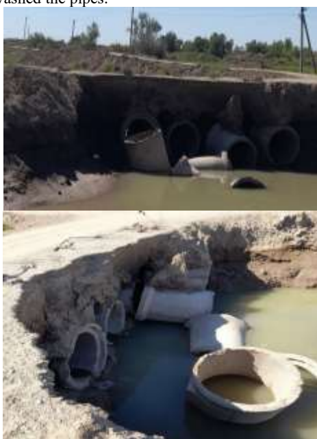
Fig. 2. Loss of load-bearing capacity of a structure as a result of soil erosion
