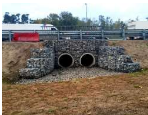
Fig. 4. Coating water pipes with gabions
