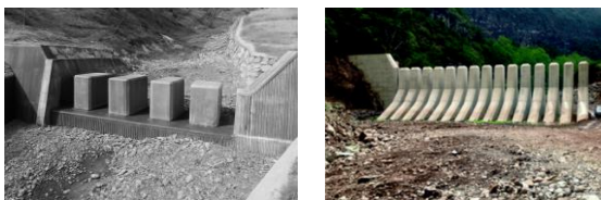
Fig. 4. Special multi-stage dams built in the direction of mudflow
