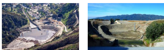
Fig. 1. Special reservoirs built in the direction of mudflow
