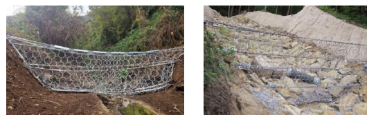
Fig. 2. Special wire mesh built in the direction of the mudflow
