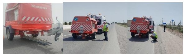
Fig. 3. Measurement of Asphalt Concrete Pavement Strength Using the Dina-4 FWD Equipment
