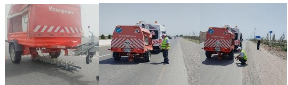
Fig. 3. Measurement of Asphalt Concrete Pavement Strength Using the Dina-4 FWD Equipment
