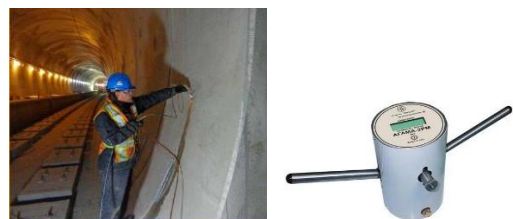
6-rasm. Tonneldagi beton qoplamaning suv o‘tkazmasligini tekshirish qurilmasi (ATAMA-2PM)
