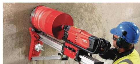
4-rasm. Betonning mustahkamligini burg'ulash usulidan bilan aniqlash
