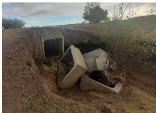
Fig. 1. Sections of the road damaged due to the loss of bearing capacity of the base
