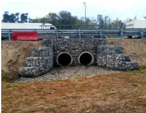
Fig. 4. Coating water pipes with gabions
