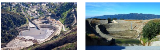
Fig. 1. Special reservoirs built in the direction of mudflow
