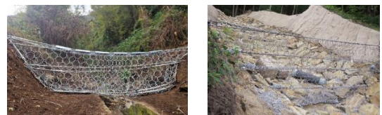
Fig. 2. Special wire mesh built in the direction of the mudflow
