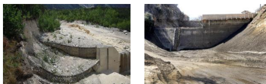
Fig. 3. Special multi-stage dams built in the direction of mudflow
